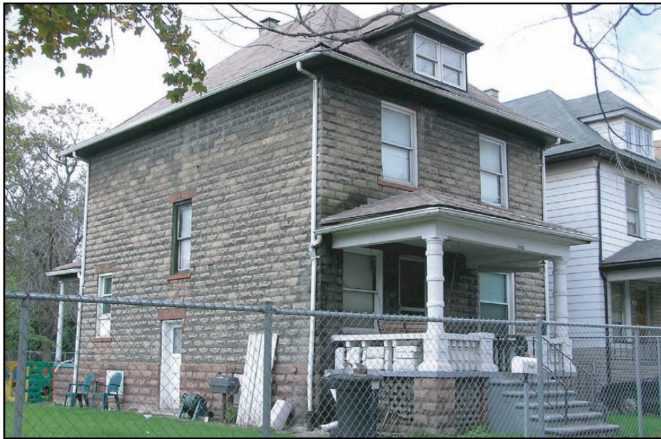
Figure 3.1.2-2. 1039 North Crawford Street
