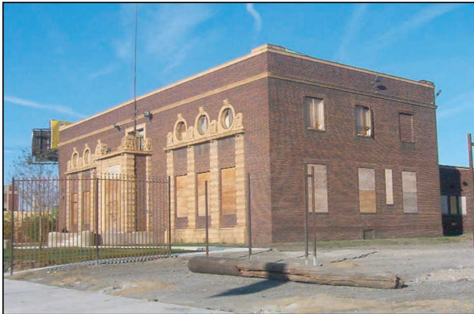
Figure 1.4.2-2. Building with Baroque Detail, 7140 West Fort Street
