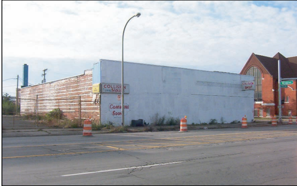
Figure 3.1.1-3. 6155 West Fort Street
