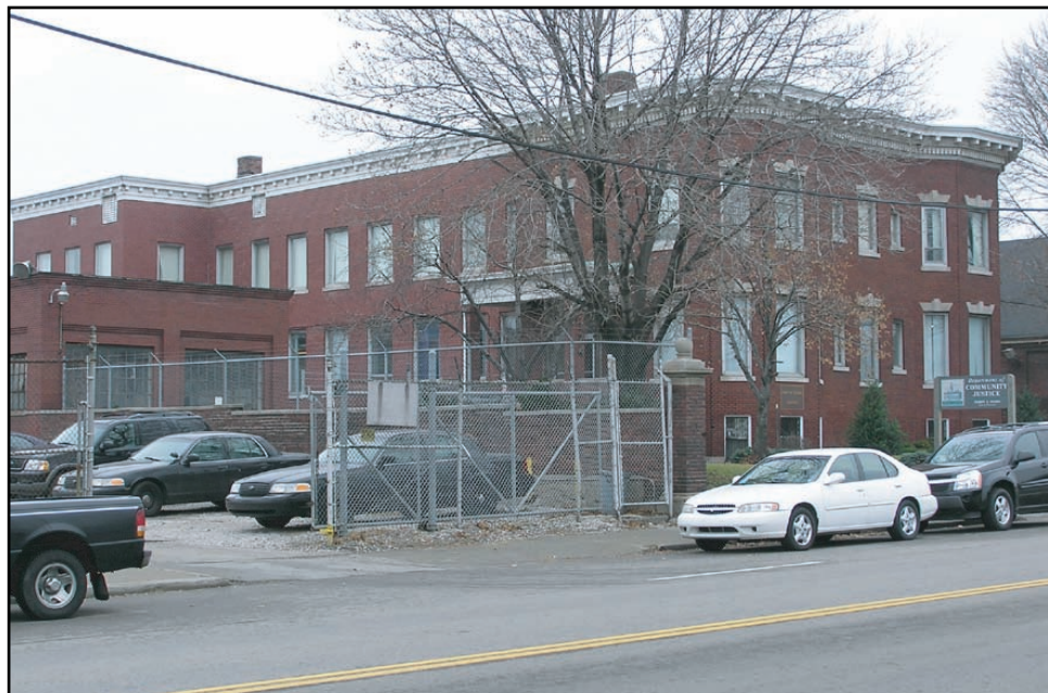
Figure 1.4.2-4. Georgian Revival Style Commercial Building, Former Detroit Copper and Brass Rolling Mills Office, 174 South Clark Street
