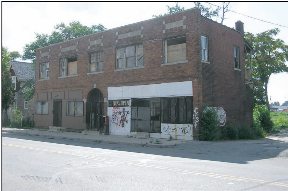
Figure 3.1.1-2. 6219 - 6123 West Lafayette Boulevard
