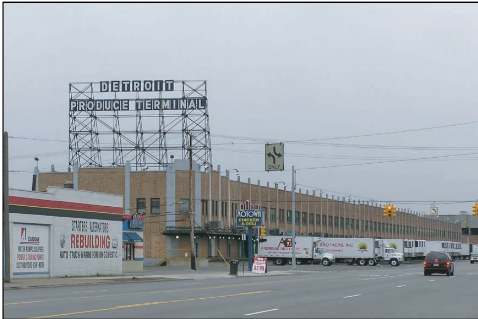
Figure 3.2.1-1. Detroit Union Produce Terminal
