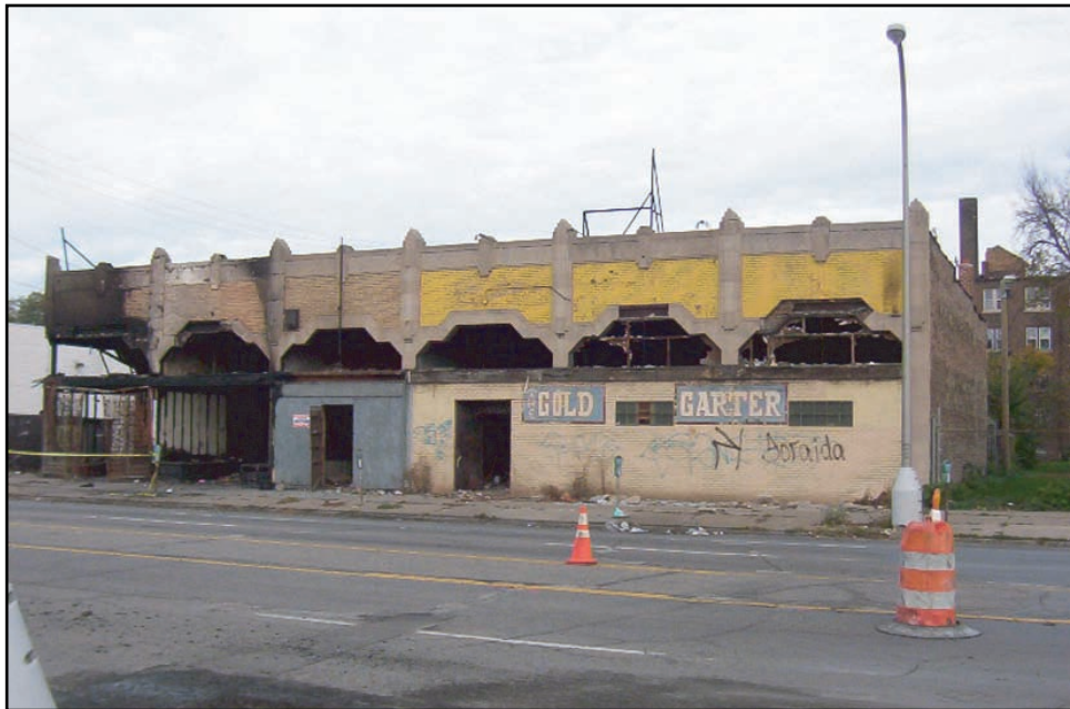
Figure 3.1.1-4. 5700 West Fort Street
